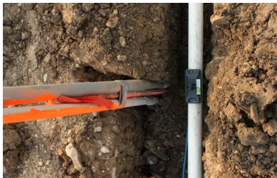
InfraMarker underground tag placed in trench over water pipe
